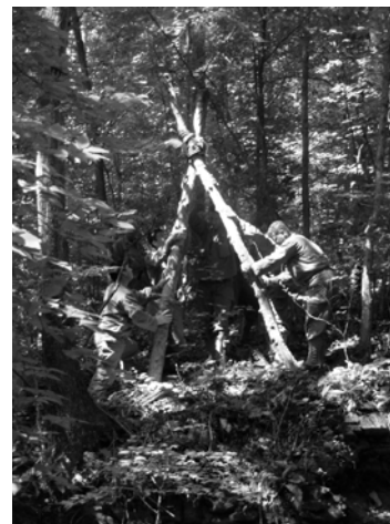
29th Ranger trainees at rigging class build an A-frame to hoist a mortar to the top of a cliff.
