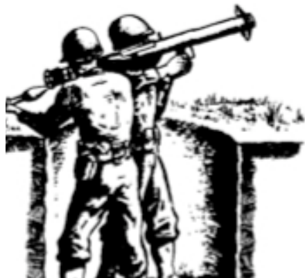
Figure 6. Pit-type emplacement for rocket launcher.
