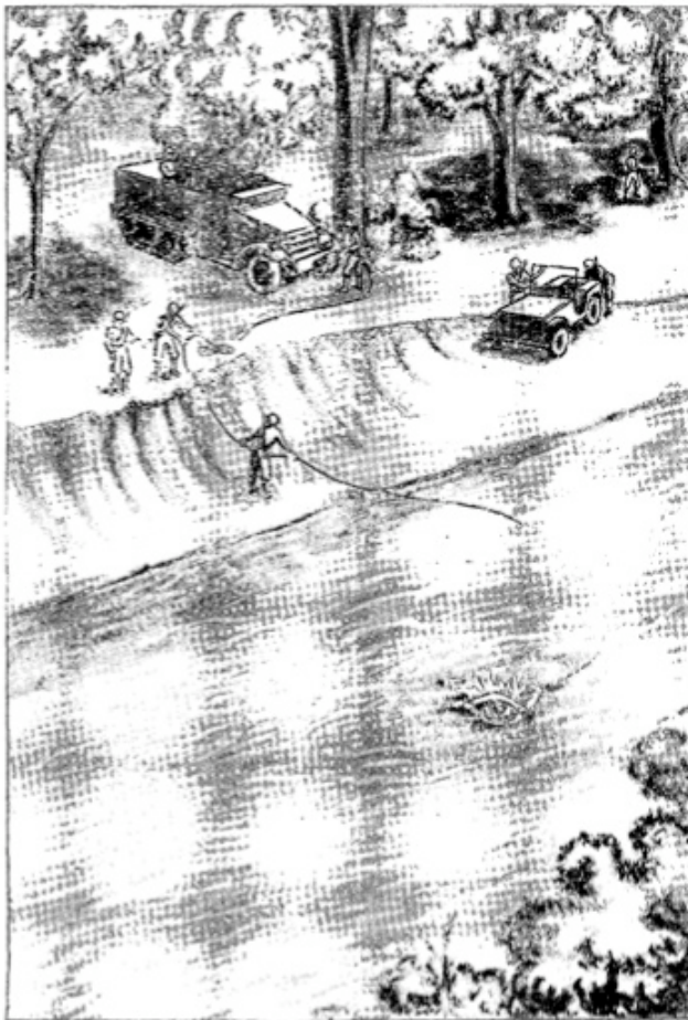
FIGURE 65.—Stringing cable from half-track winch. Winch cables are pulled across the stream by man who has crossed carrying a light line.
